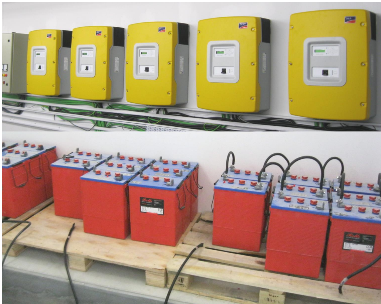
Figure 5. SMA Sunny Island inverters and the respective lead-acid batteries
