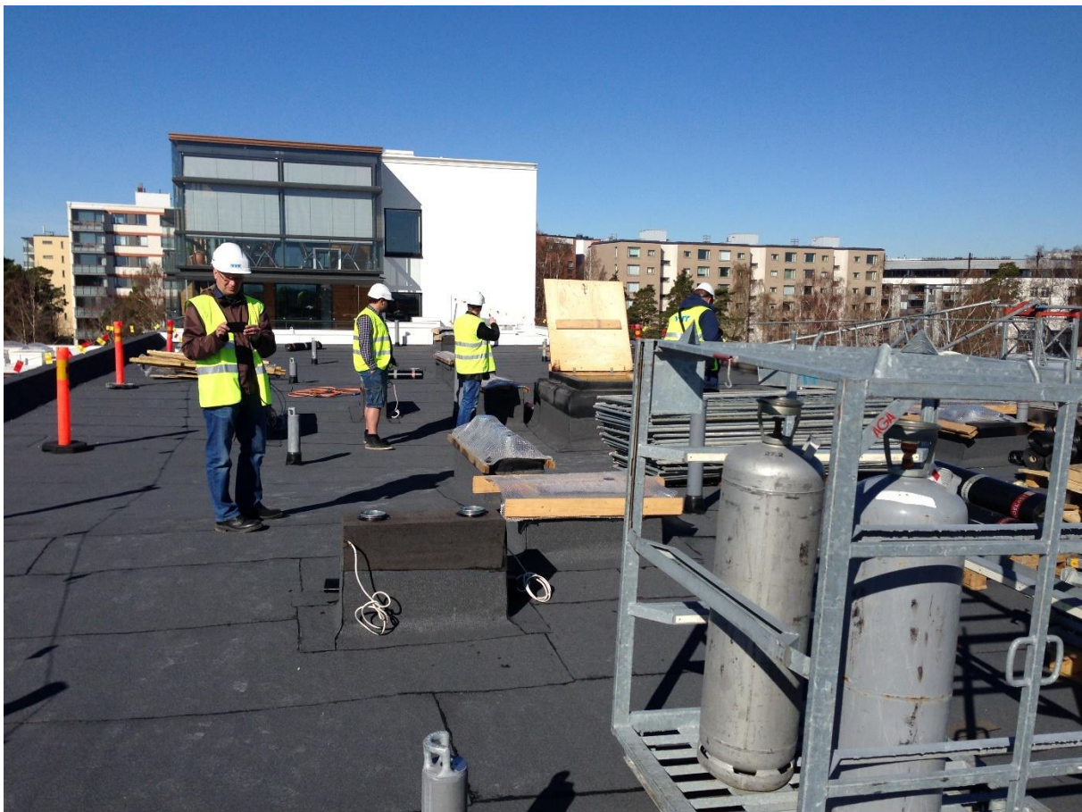
Figure 22 . Scouting for the installation location of the weather station
