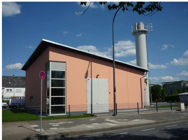
Figure 15. District heating plant Langenfeld
