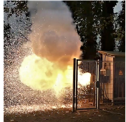
Figure 1: Investigation of high-current fault arc in the Lab at TUD (fault current = 10 kA)
